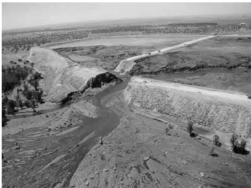
Fig. 6. Photo showing the failure of the Aznalcóllar tailings dam (Rico et al. 2008)
